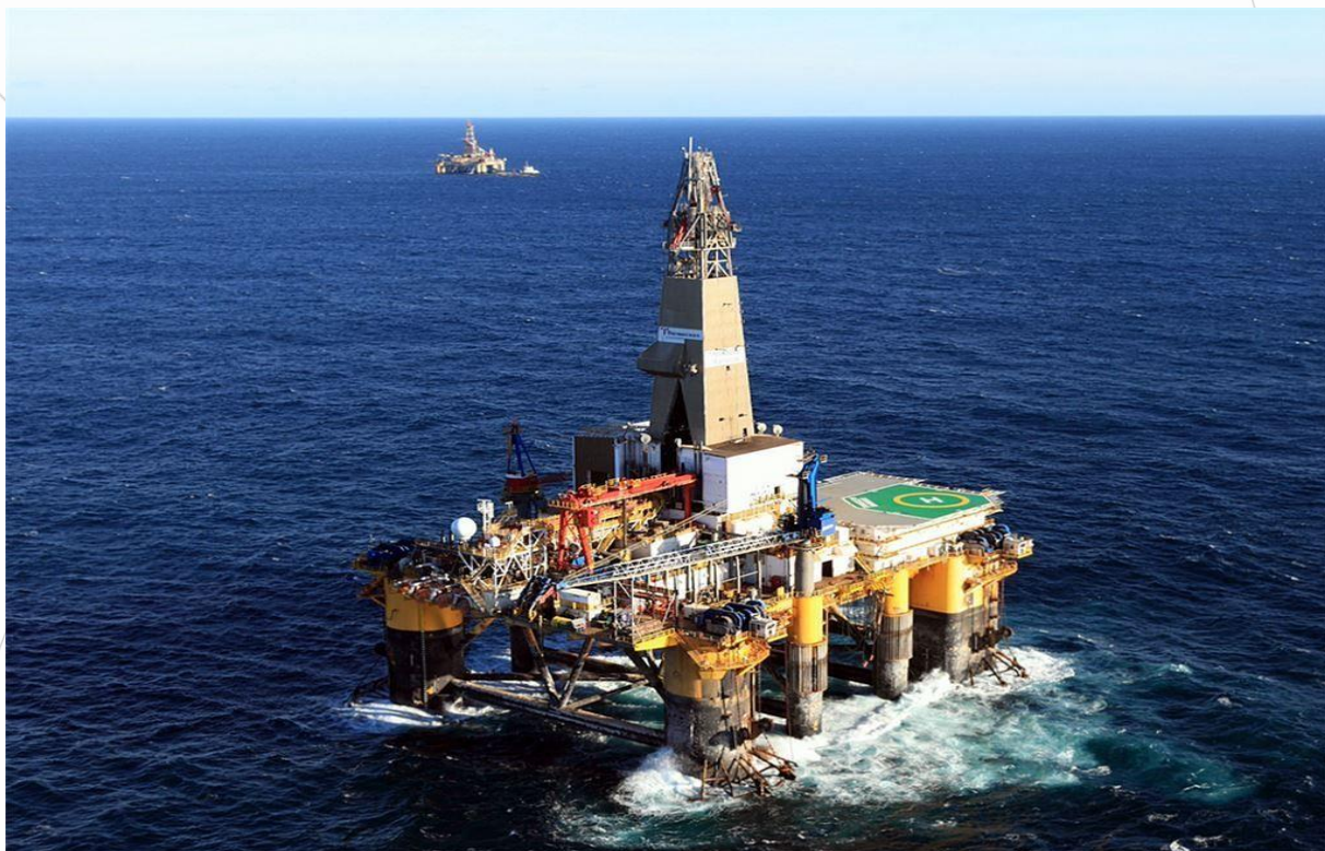
Exploratory oil drilling at the F-0 field in South Africa.
